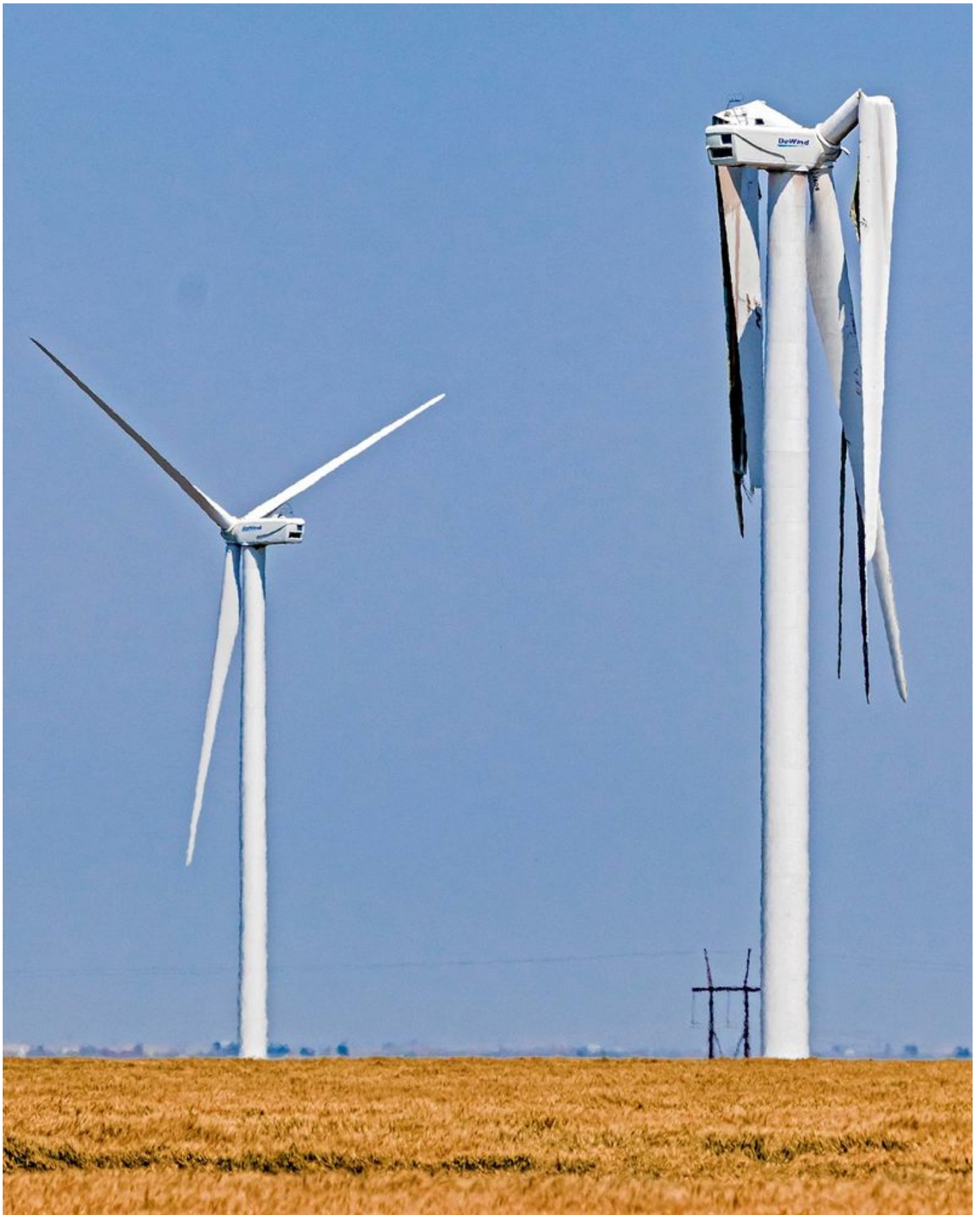
Damaged blades hang from a wind turbine near Guymon, Oklahoma, in 2021. Photographer: Chris Landsberger/The Oklahoman
